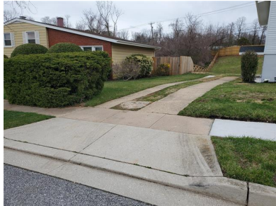
Driveway (Concrete/ See Comments)
