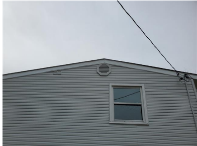
Attic Ventilation (Gable Vents)
