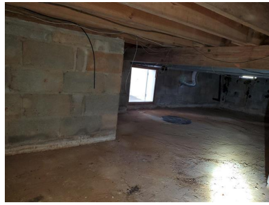
Foundation (Crawl Space/ Concrete Block)
