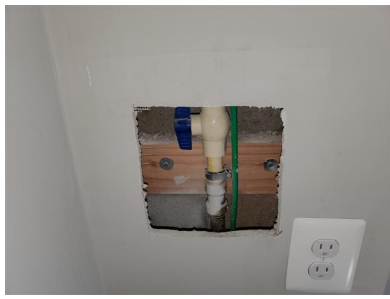
Water Service Pipe (Copper Observed)
