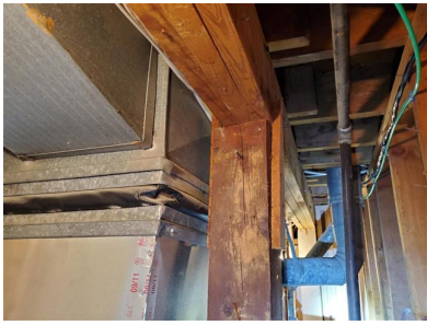
Beam (Basement/ Wood/ Built-Up Beam)
