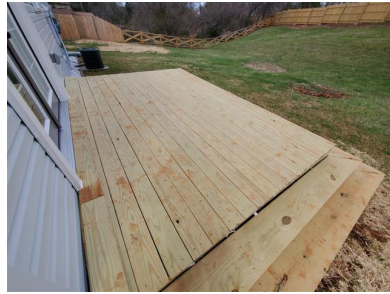
Rear Deck (Wood Decking)
