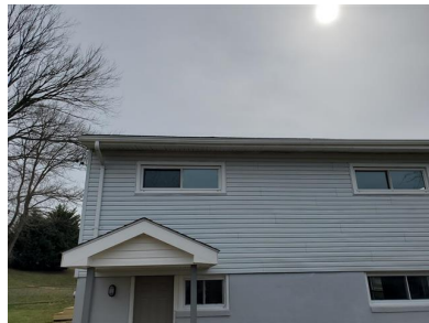
Gutters (Properly Secured/ Sloped Toward Downspouts)
