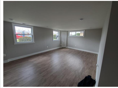
Foundation (Basement/ Finished Areas Limit Inspection)
