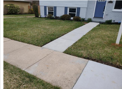
Walks (Concrete/ No Apparent Trip Concerns)
