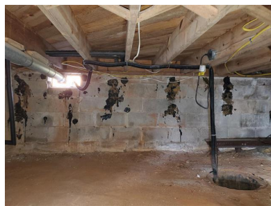
Foundation (Crawl Space/ Concrete Block)
