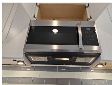
Ventilation System (Recirculating)
