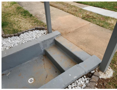
Left Rear Basement Stairwell Steps (Concrete)
