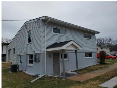
Gutters and Downspouts (Aluminum)
