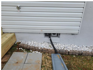
Crawl Space Ventilation (Manual Crawl Space Vents)
