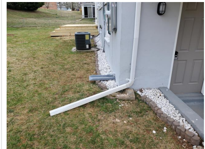
Downspout Extensions (Good/ Move Water Away from Foundation)
