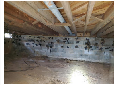
Foundation (Crawl Space/ Concrete Block)
