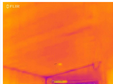
Thermal IR Scan (No Evidence of Water Intrusion Through Roof)
