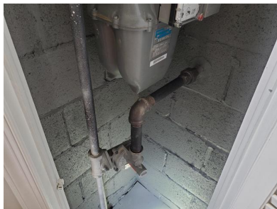
Foundation (Basement/ Concrete Block)
