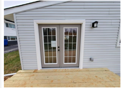
Rear Deck Entrance Door (Metal Clad Wood/ Insulated Glass)
