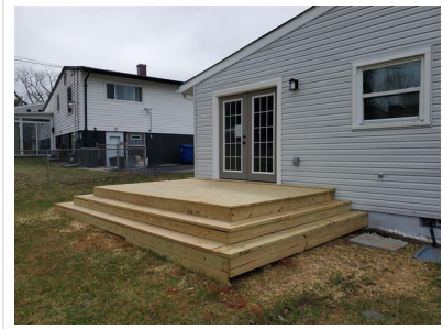
Rear Deck (Wood/ See Comments)
