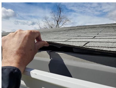
Visible Flashing (Looks Good)
