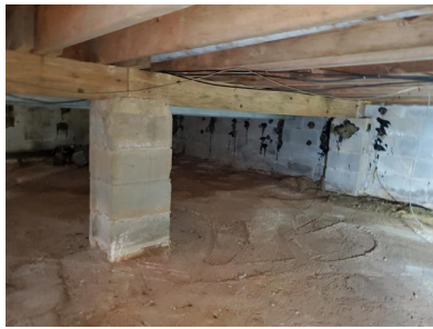
Piers (Crawl Space/ Concrete Block)
