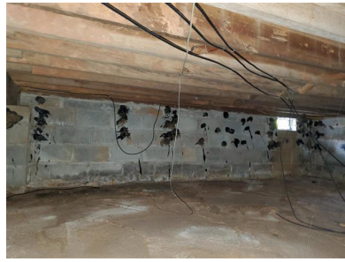
Foundation (Crawl Space/ Concrete Block)
