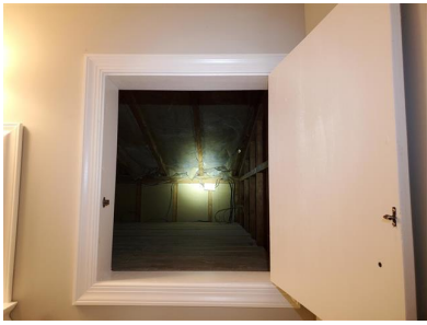
Attic Access (Door/ Second Floor Hallway Bathroom)
