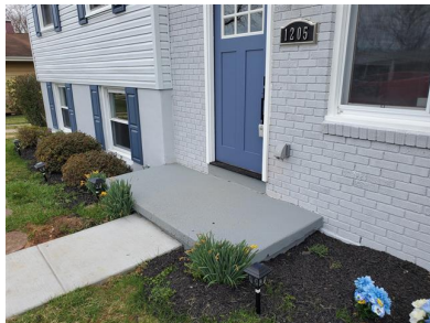
Front Entrance Stoop (Concrete/ Open/ Concrete in Good Condition)
