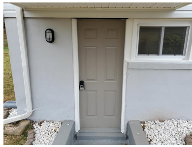
Left Rear Basement Stairwell Entrance Door (Metal Clad Wood)
