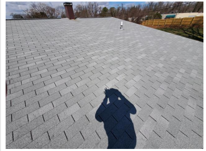
Roof Covering (3-Tab Asphalt Shingle)
