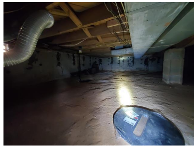
Crawl Space Photos (No Evidence of Abnormal Water Intrusion)
