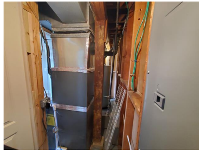
Posts (Basement/ Wood)
