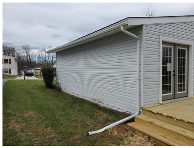
Gutters and Downspouts (Aluminum)
