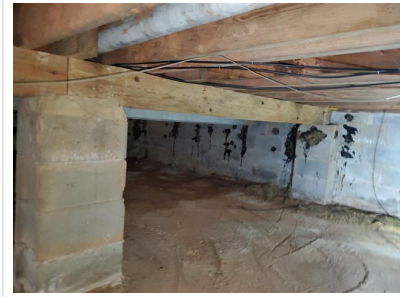
Beam (Crawl Space/ Wood/ Built-Up Beam)
