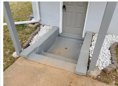
Left Rear Basement Stairwell Retaining Walls (Concrete Block/ Monitor Previous Repairs)
