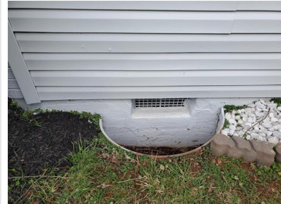
Crawl Space Ventilation (Manual Crawl Space Vents)
