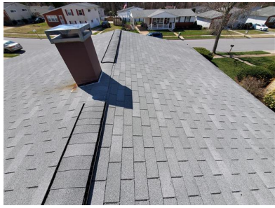
Roof Covering (3-Tab Asphalt Shingle)
