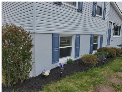
Foundation (Exterior/ Parged Concrete Block)
