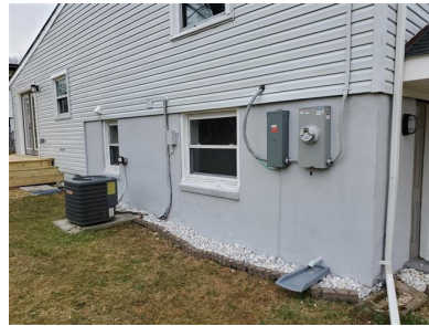
Foundation (Exterior/ Parged Concrete Block)
