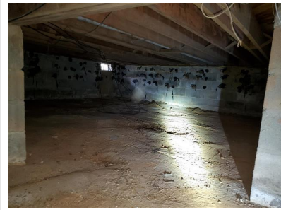
Crawl Space Photos (No Evidence of Abnormal Water Intrusion)
