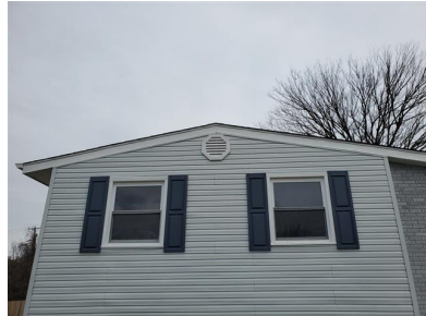
Attic Ventilation (Gable Vents)
