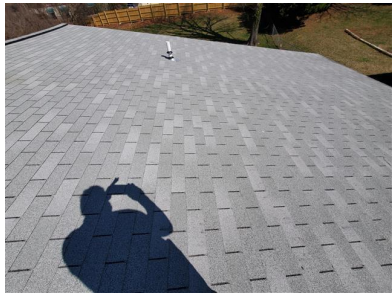
Roof Covering (3-Tab Asphalt Shingle)
