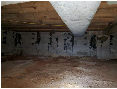
Foundation (Crawl Space/ Concrete Block)
