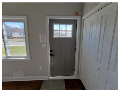
2.6 Item 4 (Picture) Door Binding Perspective Photo (Front Entrance Door)
