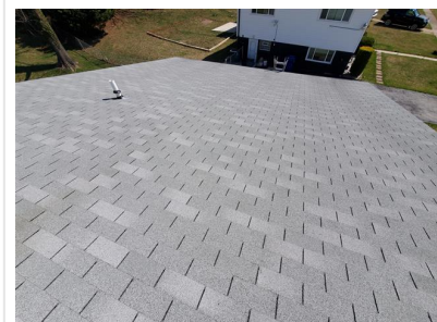
Roof Covering (3-Tab Asphalt Shingle)
