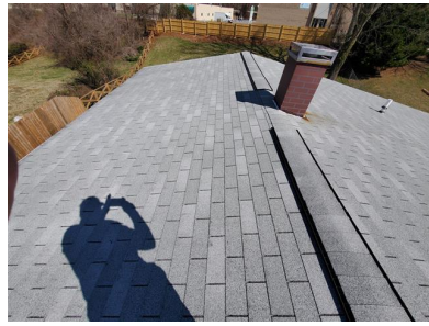
Roof Covering (3-Tab Asphalt Shingle)
