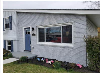
Siding 1 (Brick Veneer)
