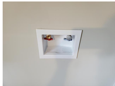
13.6 Item 1 (Picture) Standpipe Not Observed (Clothes Washer Connections Box)
