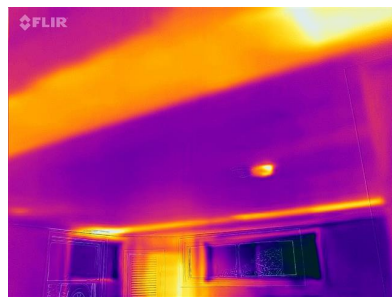
Thermal IR Scan (No Evidence of Plumbing Leaks Between Floors)
