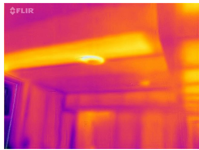
Thermal IR Scan (No Evidence of Plumbing Leaks Between Floors)
