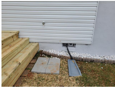
Foundation (Exterior/ Parged Concrete Block)
