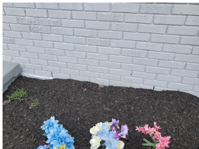
Brick Veneer Weep Holes (Do Not Fill)
