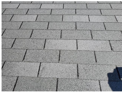
Roof Covering (3-Tab Asphalt Shingle)
