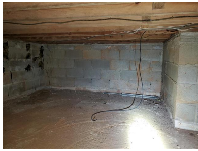
Foundation (Crawl Space/ Concrete Block)
