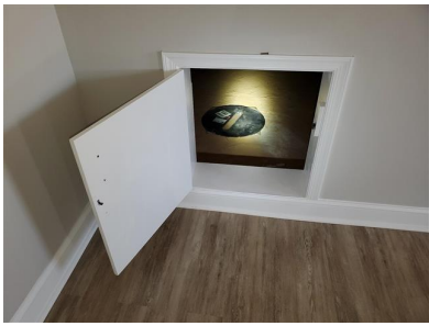
Crawl Space Access (Door/ Basement Hallway)
