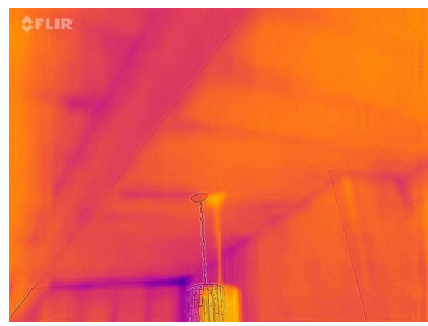
Thermal IR Scan (No Evidence of Water Intrusion Through Roof)
