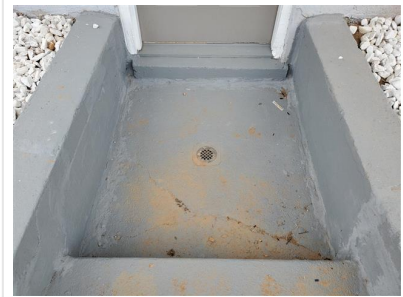
Surface Drain (Left Rear Basement Stairwell)
