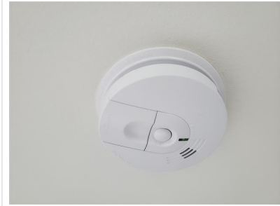
Bedroom Smoke Detectors (Acceptable)
