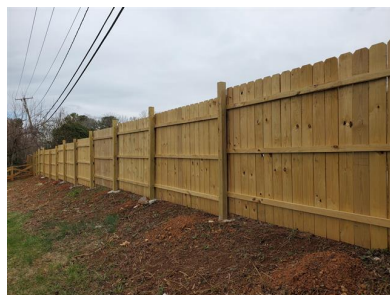
Rear Fence (Wood/ See Comments)
