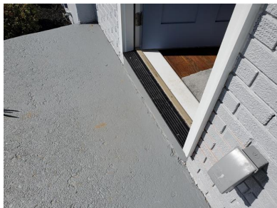
12.5 Item 4 (Picture) Patched Drill Holes/ Previous Termite Treatment (Front Stoop)
