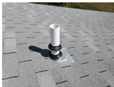
Visible Flashing (Looks Good)
