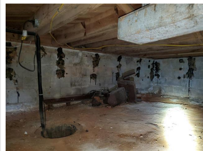
Foundation (Crawl Space/ Concrete Block)
