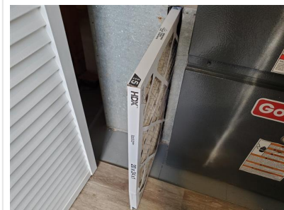
Air Filter Size (20x24x1) and Air Flow Direction (Arrow Toward Furnace)
