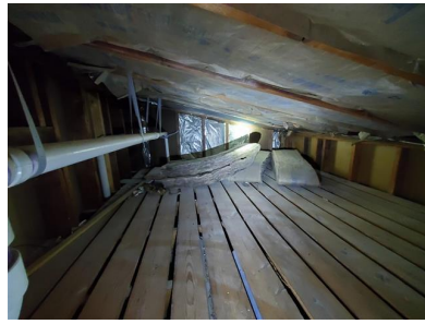
Attic (No Water Stains or Evidence of Water Intrusion)
