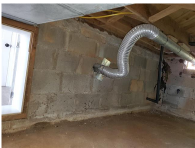
Foundation (Crawl Space/ Concrete Block)
