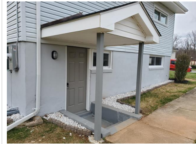
Foundation (Exterior/ Parged Concrete Block)
