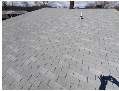
Roof Covering (3-Tab Asphalt Shingle)
