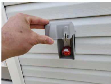
Exterior Receptacles (Weather Covers/ GFCI Protection/ Resets at Receptacles)
