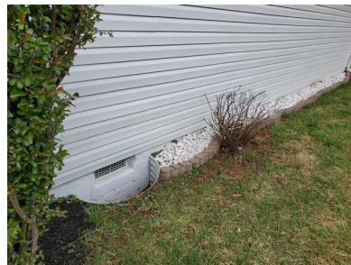
Foundation (Exterior/ Parged Concrete Block)
